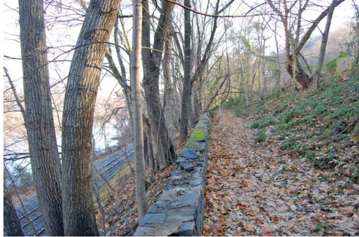
Stone parapet along abandoned River Road
