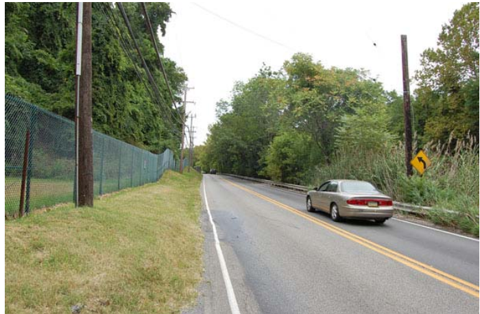
River Road north of Blue Route viaduct
